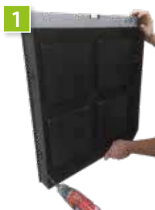
▪ Attach back frame to wall
